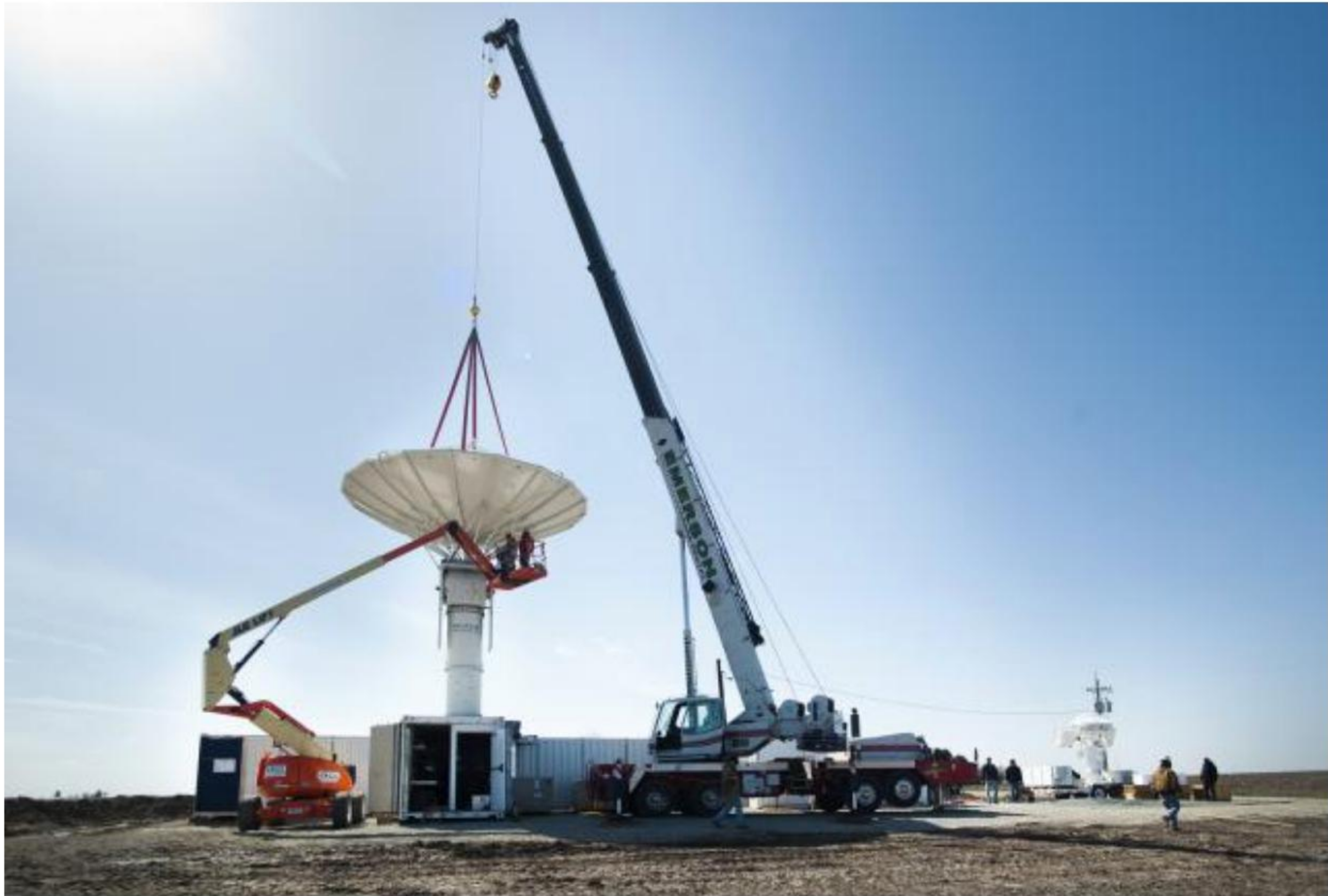
A large crane drops the NPOL antenna into place. The NPOL radar is located in eastern Iowa near Waterloo for the IFloodS campaign (May 1-June 15). Photo by Aneta Goska, Iowa Flood Center.
