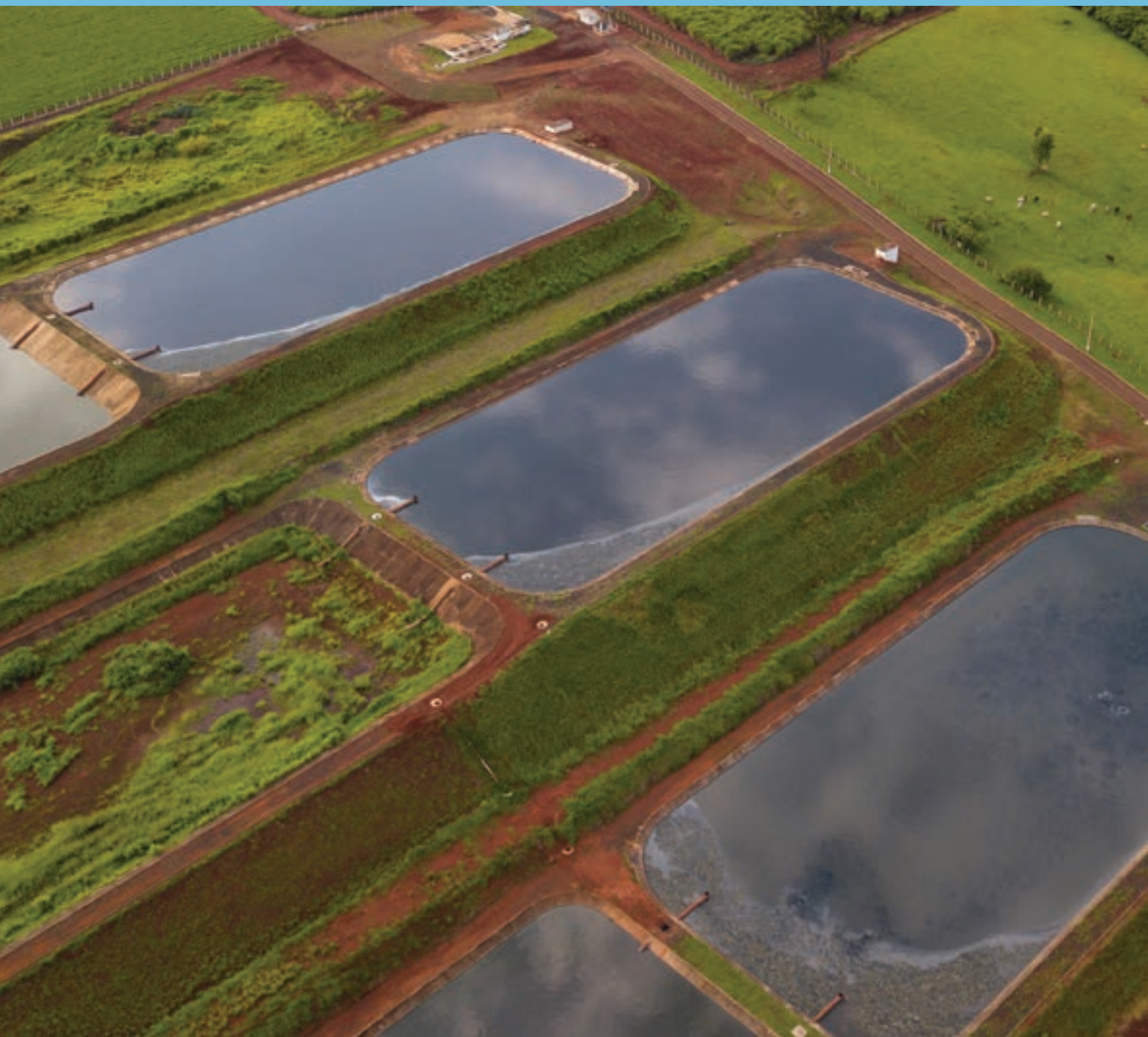
Aerial view of a sewage treatment facility.
