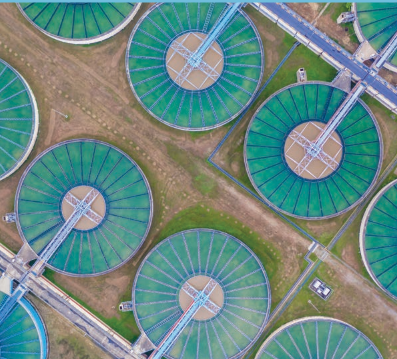
Aerial view of a water treatment plant.
